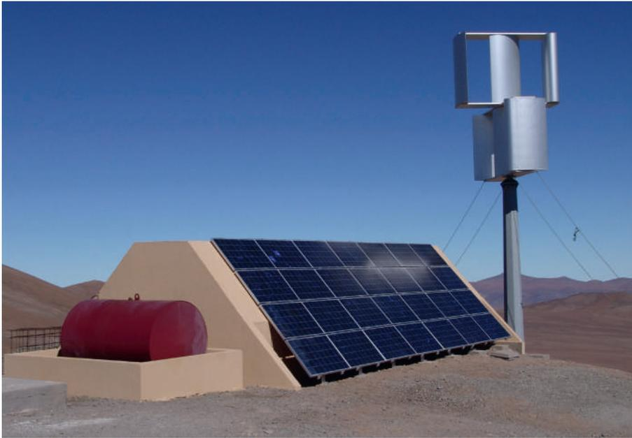
**Fig. 4.** Battery house with solar panels, windmill and tank for the back-up generator (August 15, 2008).
